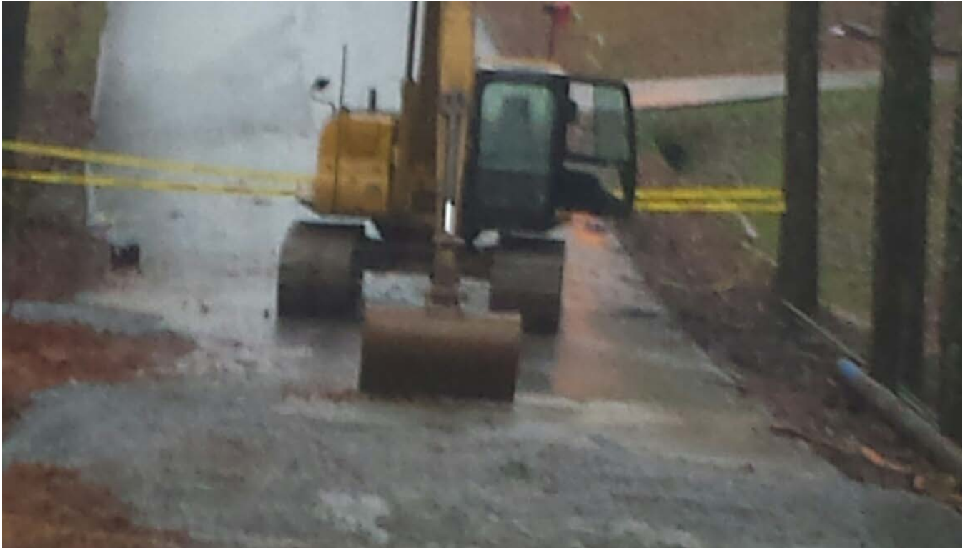
Photo 1: Canterbury Lane is being repaired for road reopening.
